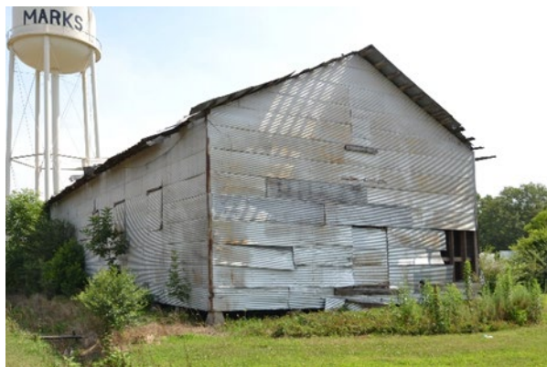
Above is the seed house associated with the Self Gin, which is non-extant.
