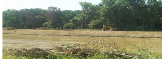
Construction along the bank of the Tallahatchie River Item 6B near Phillip, MS
